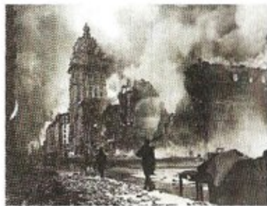
After the earthquake
